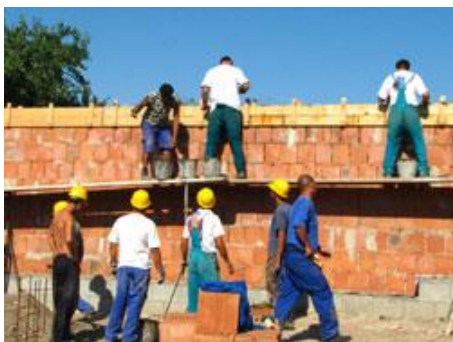
Finishing off the walls of the Carpenters' Workshop
